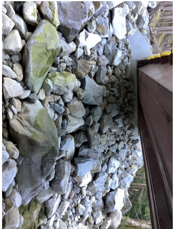
Left Bank Abutment when facing downstream
